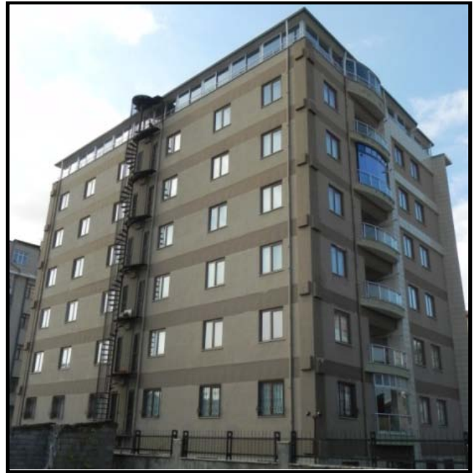
Fotoğraf/Picture 72 – Ard-germeli Binada Halihazır Görünüş / The Current View of the Building with Post-Tensioned Connections
