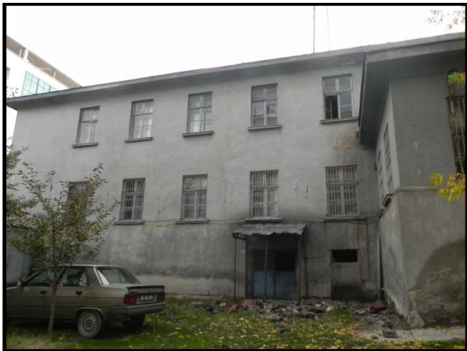
Fotoğraf/Picture 29 – Bina Yan Cephesi / Side View of the Building
