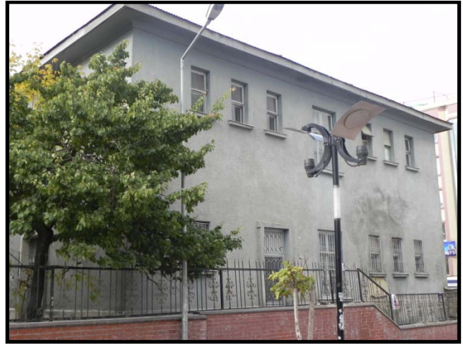
Fotoğraf/Picture 28 – Bina Yan Cephesi / Side View of the Building
