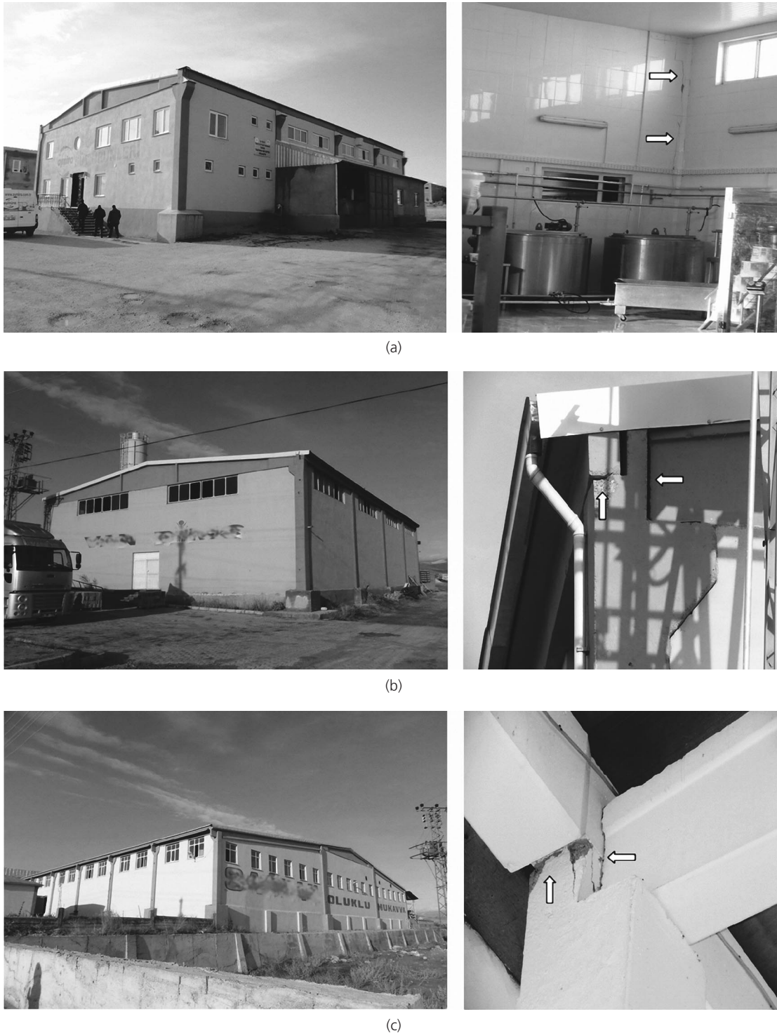
Figure 5. Examples of precast concrete facilities having light damage in the city industrial zone (CIZ) of Van city
