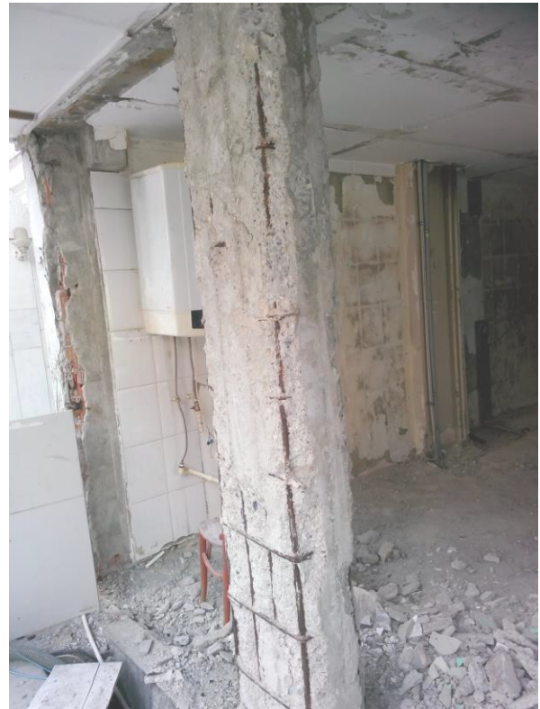
Fig.2 - Corrosion Damage on Columns
