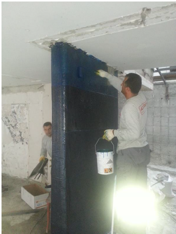
Fig.7 – CFRP Application on Shear Walls
