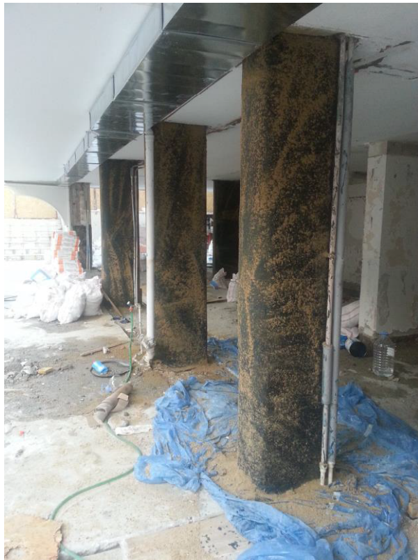
Fig.9 – Sand Cover for Better Plastering
