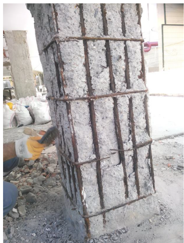
Fig.4 – Cleaning on Corner Column
