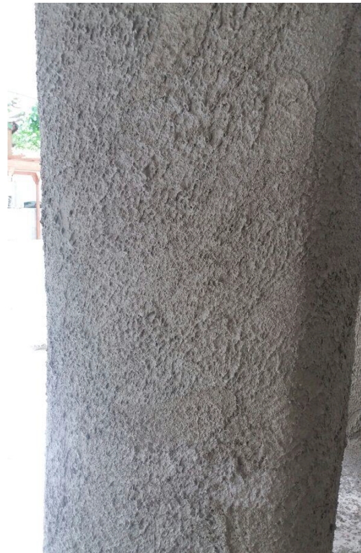
Fig.10 – Plastering Against Fire
