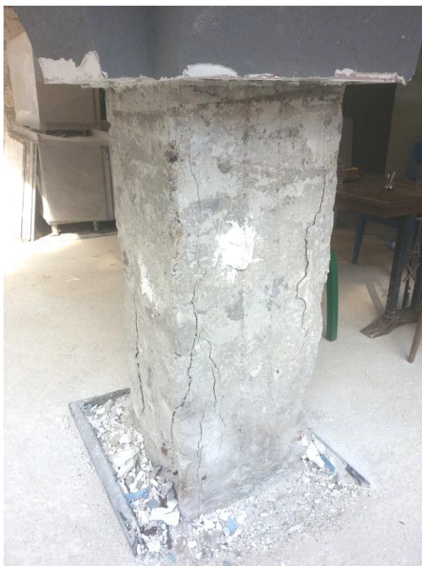
Fig.3 – Cracks on Corner Column
