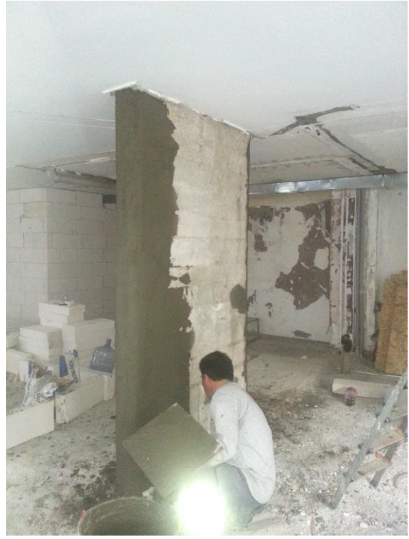
Fig.6 – Restoring the Original Cross-Section
