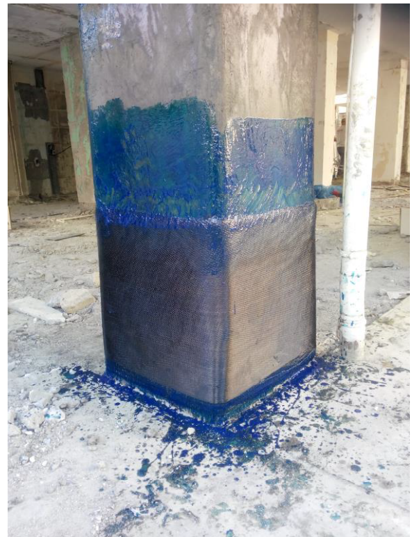
Fig.8 – CFRP Application on Corner Columns
