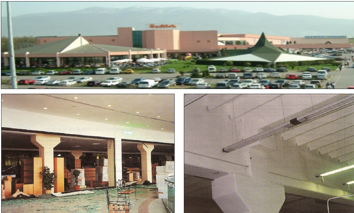
Figure 9 – Performance of a Shopping Mall after 1999 Kocaeli Earthquake [12]
