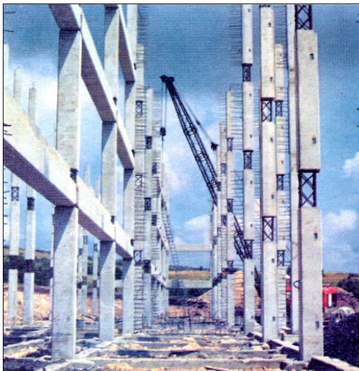
Figure 5 – Precast Multi-Storey Building during Construction and After 2003 Bingol Earthquake [9]
