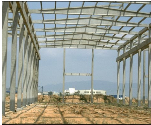
Figure 2 – Industrial Building under Construction in Adana in 1998 [6]
