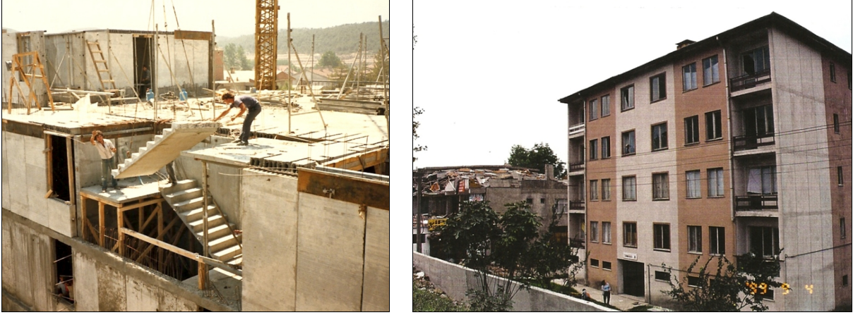
Figure 6 – Precast Multi-Storey Wall System Building during Construction and After 1999 Kocaeli EQ. [10]
